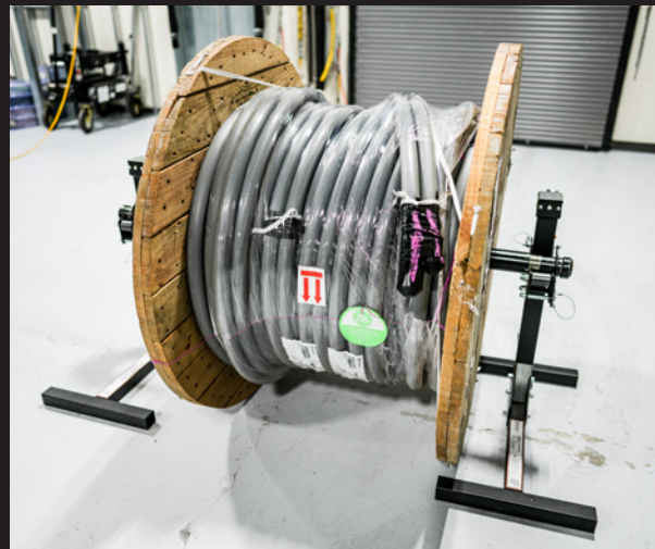
TWO CONDUITS ON A SINGLE REEL
