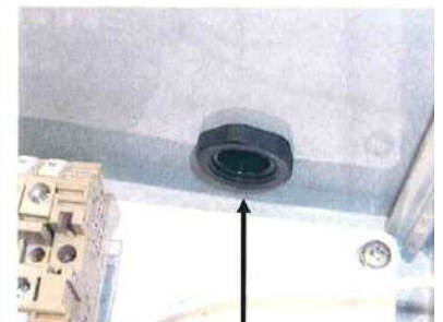
Strain relief bushing nut on inside of enclosure.
