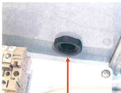
Strain relief bushing nut on inside of enclosure.
